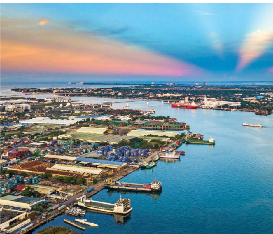
A new international container terminal is being constructed at the port of Cebu
