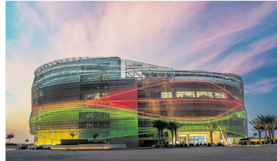
State-of-the-art new office headquarters building for Omantel in Muscat.
