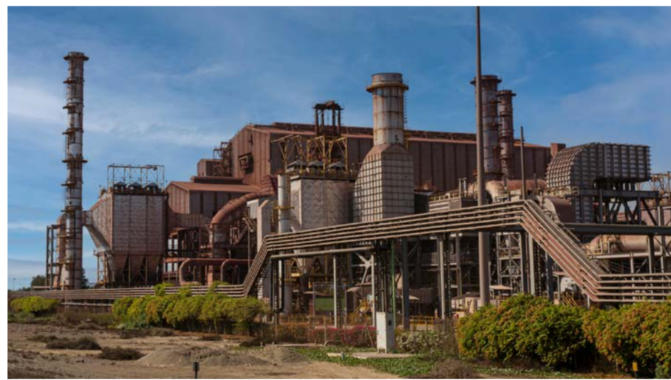
Iron factory in Sohar Port, Oman.
