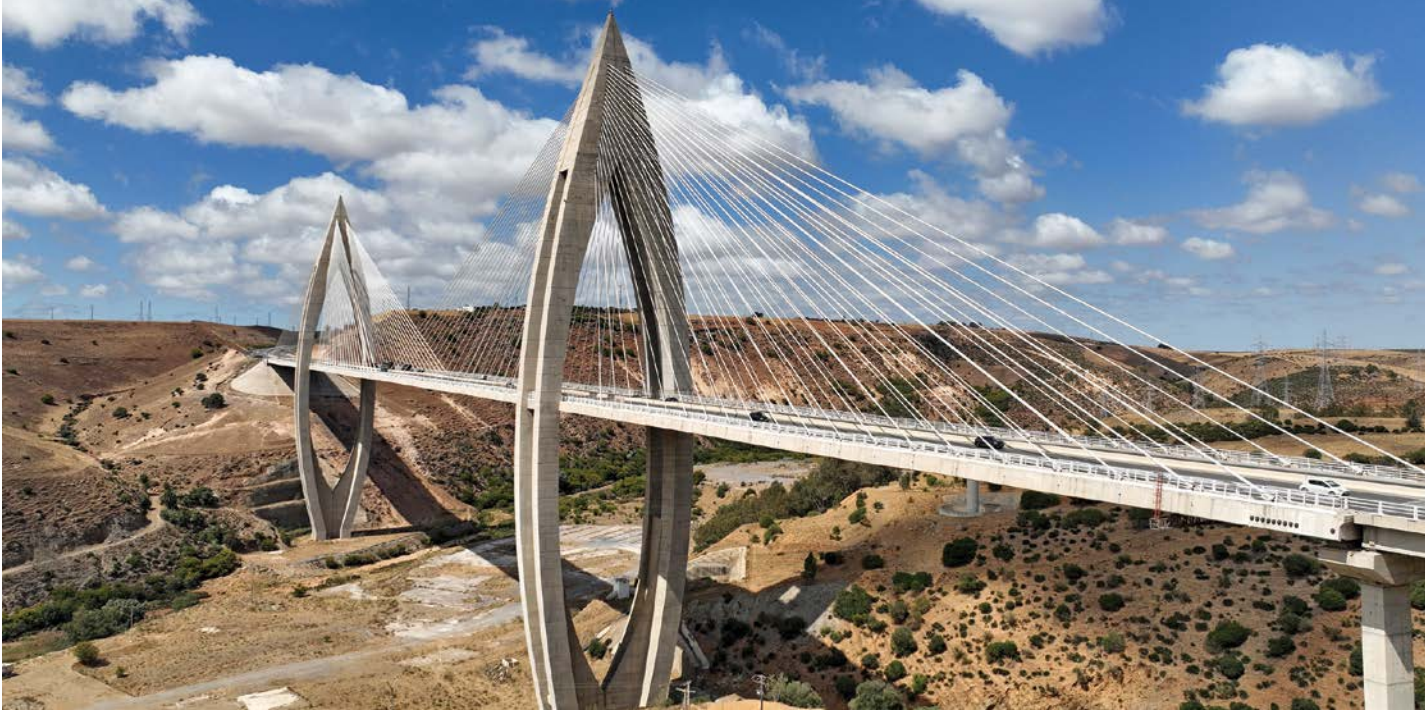
Opened in 2016, Mohammed VI Bridge connects the cities of Rabat and Salé, and is the longest cable-stayed bridge in Africa
