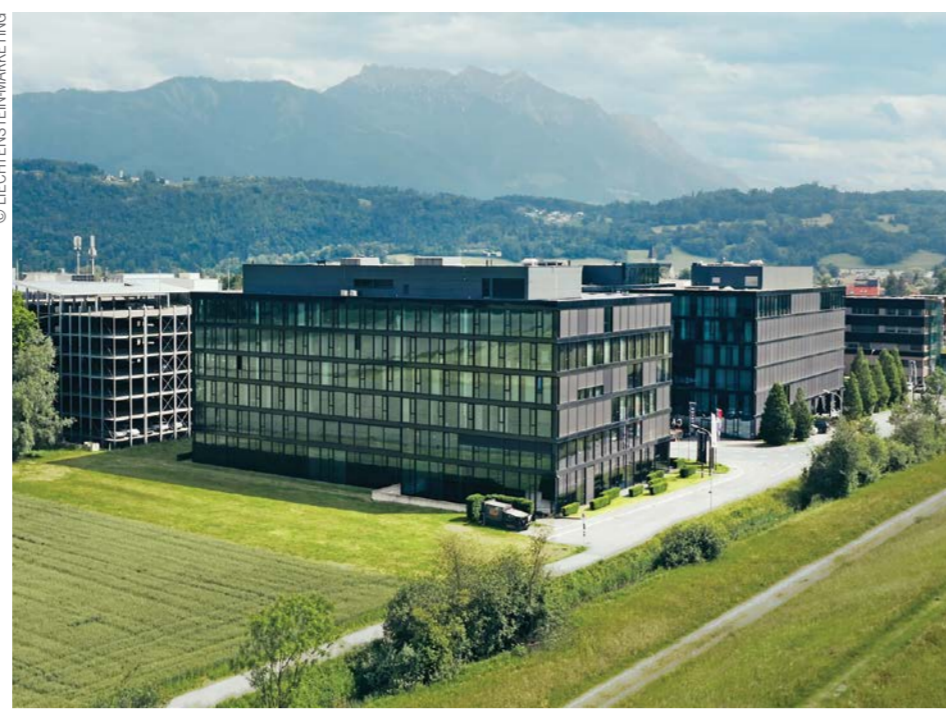
Modern and comfortable offices with spectacular mountain views inspire workers
