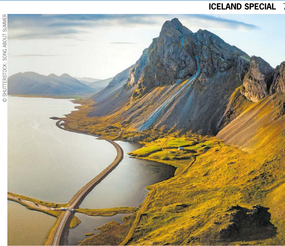
Major investments are going into the country's roads.
