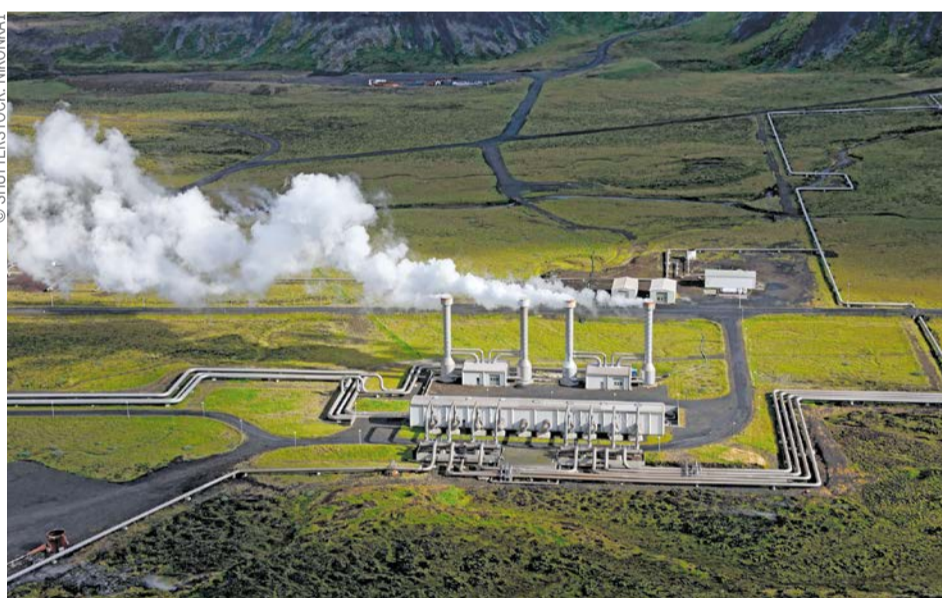
Construction of the Nesjavellir Geothermal Power Station began in 1987.
