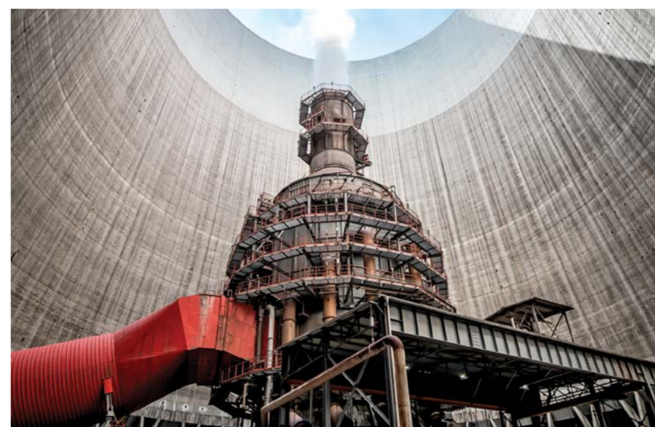
A Heller-Forgó cooling tower at Mátra Power Plant
