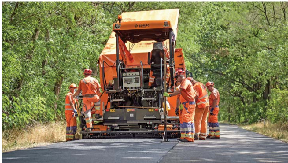
Hungarian Public Roads operates and maintains nearly 20,000 miles of national roads
