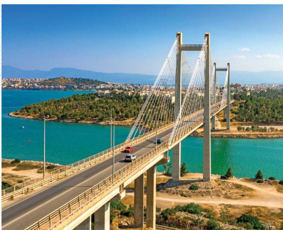
The modern suspension bridge to Evia or Euboea, Greece's second-largest island
