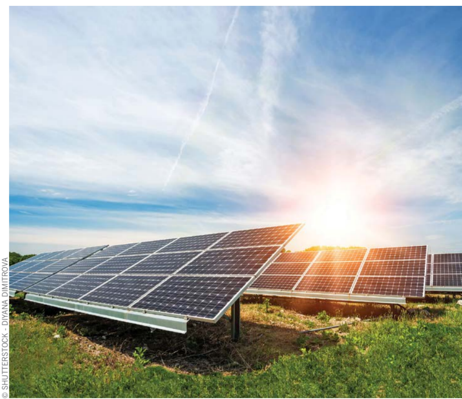
Belize is exploring the possibility of further utilizing solar energy
