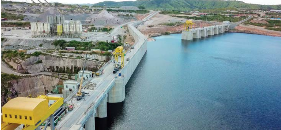
Angola is a world leader in hydroelectricity.
