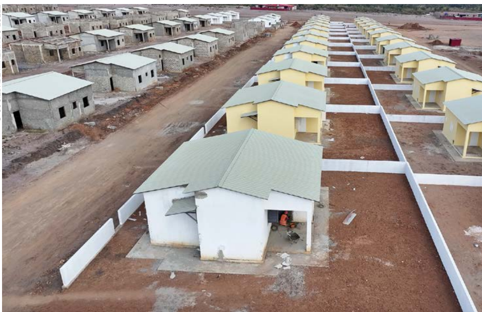
Sociedade Mineira do Luele is building 350 homes for its local community.
