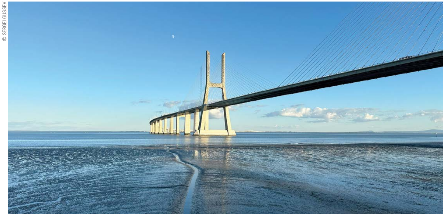
The Vasco de Gama Bridge in Lisbon, an enduring symbol of Portugal's progress and connectivity.
