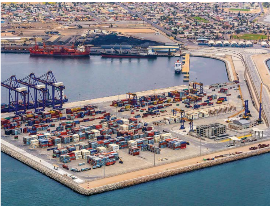
Modern logistics infrastructure at Walvis Bay has made the nation an import/export hub.
