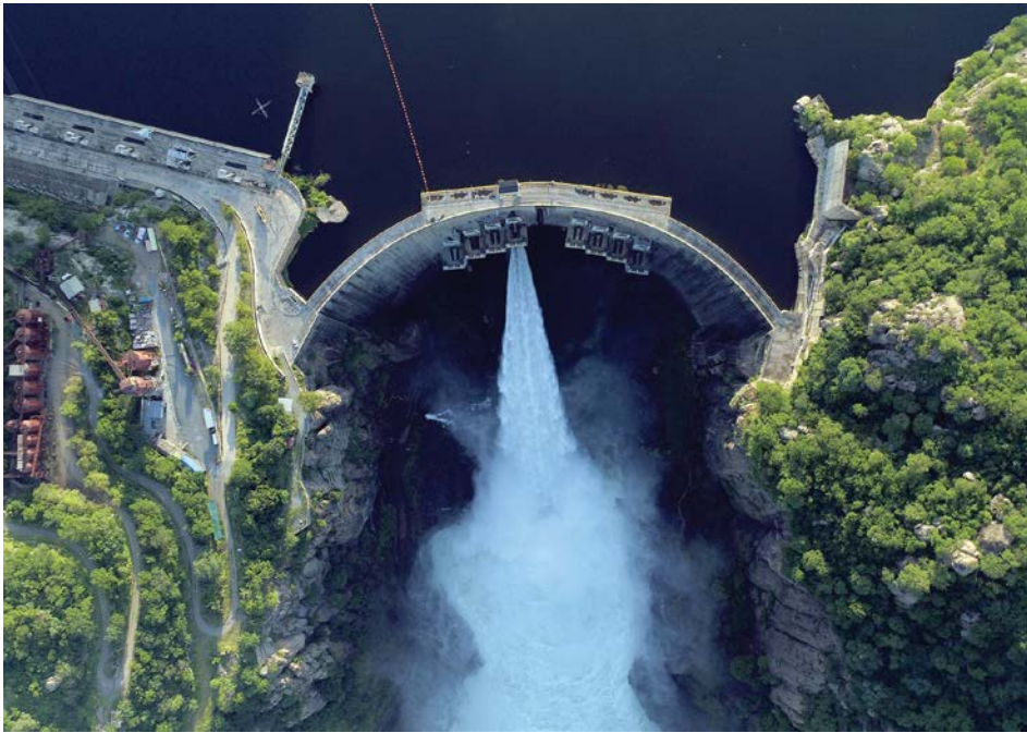
The Cahora Bassa Dam is the largest hydroelectric power plant in Southern Africa.
