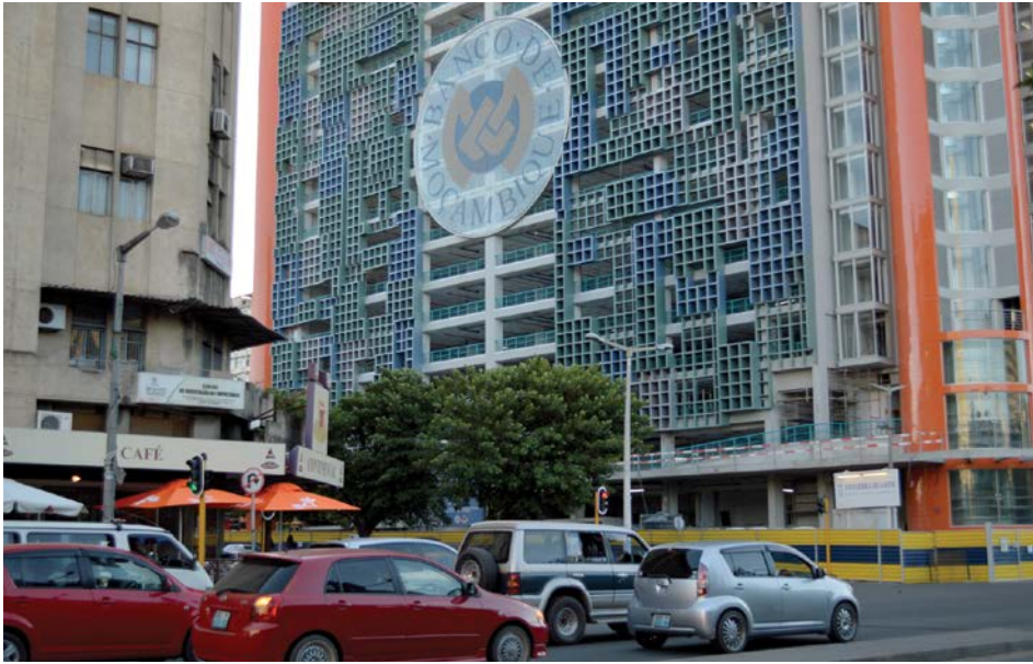
The Central Bank oversees Mozambique's highly competitive banking sector.
