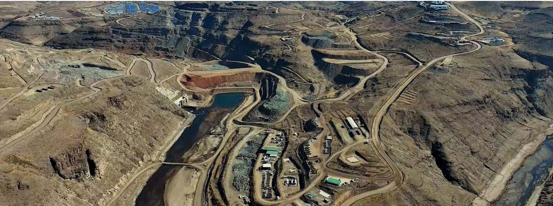
The second phase of the Lesotho Highlands Water Project requires huge amounts of infrastructure development.
