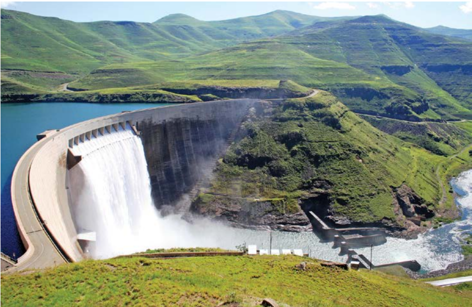
Katse Dam is Africa’s second largest double-curvature arch dam.
