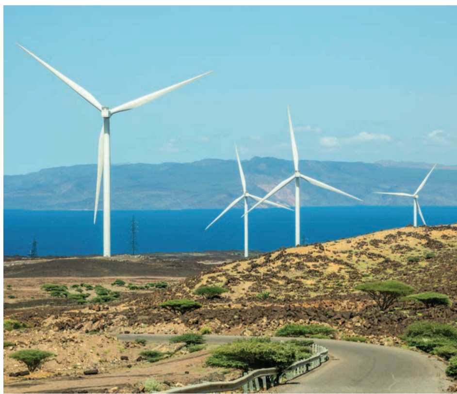
The wind turbines of the Ghoubet wind power station generate 60 MW of electricity
