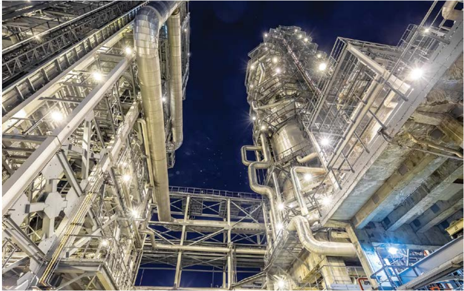
Bolivia has three primary refining facilities all operated by YPFB.
