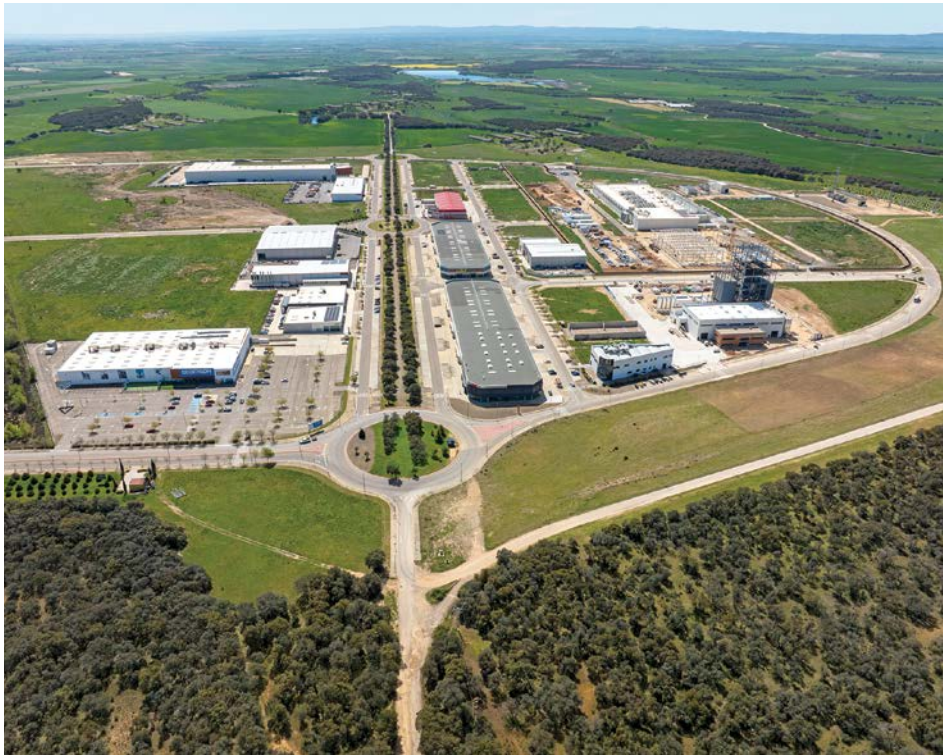
Plaza Logistics Park is one of the largest intermodal logistics hubs in Europe
