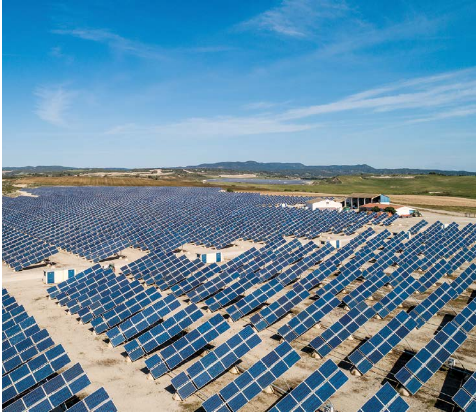
Zuera photovoltaic plant (20 megawatts)
